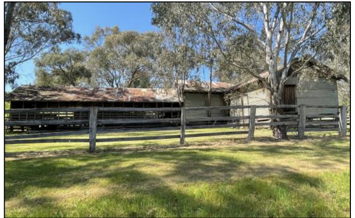
Glen: Farm shed.
